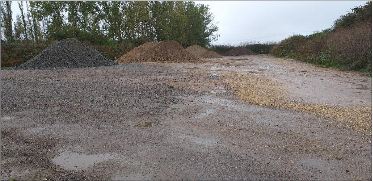
Looking south-east across Area B. Stockpiles of brick crush, concrete crush and granite are present.
