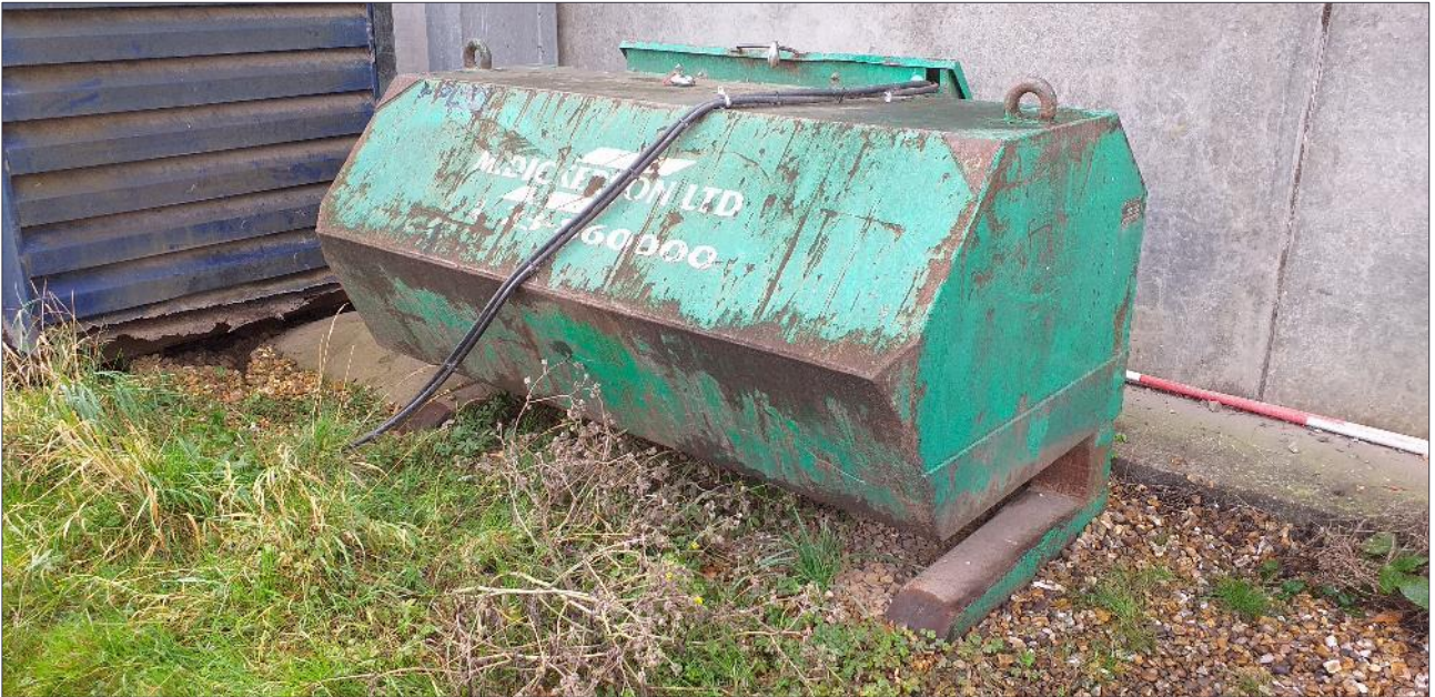
Diesel fuel tank adjacent to the north-west corner of the WRW used to fuel the plastic wrapping system.
